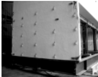
6. Crossbow Civil & Structural Solution
