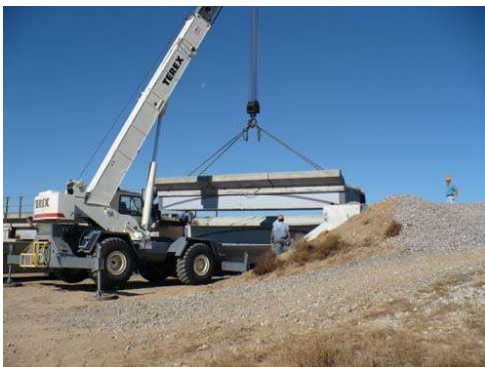
Setting HCB Unit on Bridge Substructure
